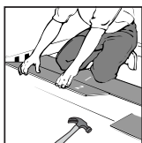
[7] It's easier to assemble if you kneel on top of the planks and use a pulling motion to insert.
